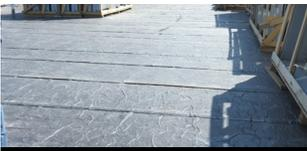
Moisture has appeared to have created wrinkles and bubbles on this fully adhered vapor barrier installation.
